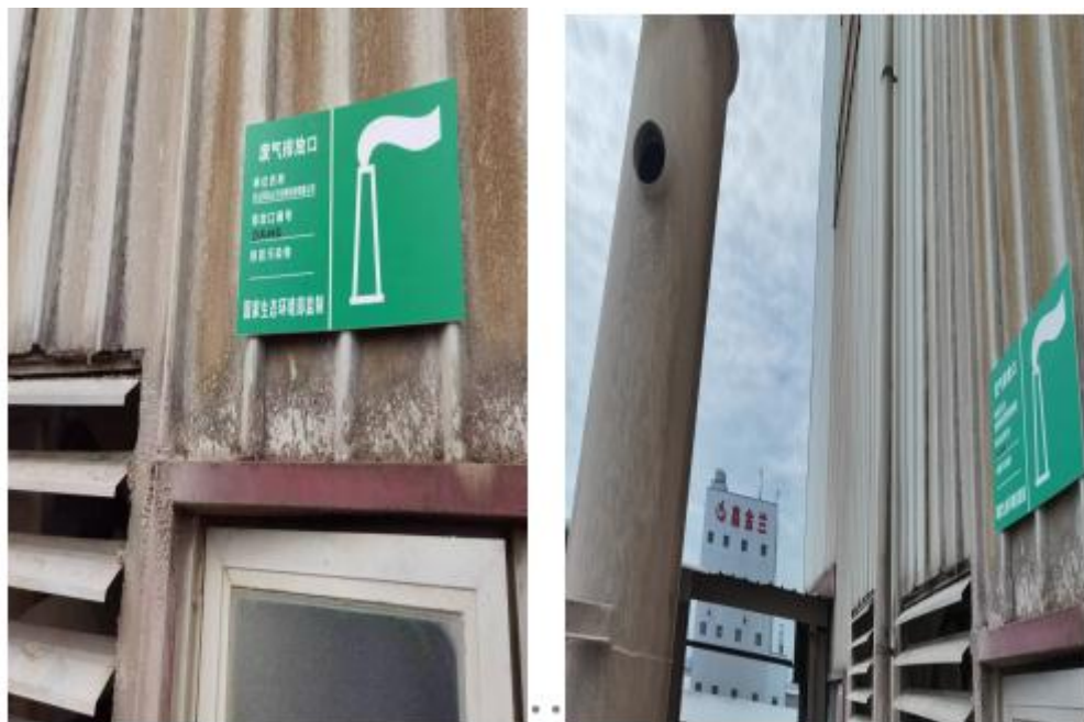
DA002.....DA002 废气治理设备
