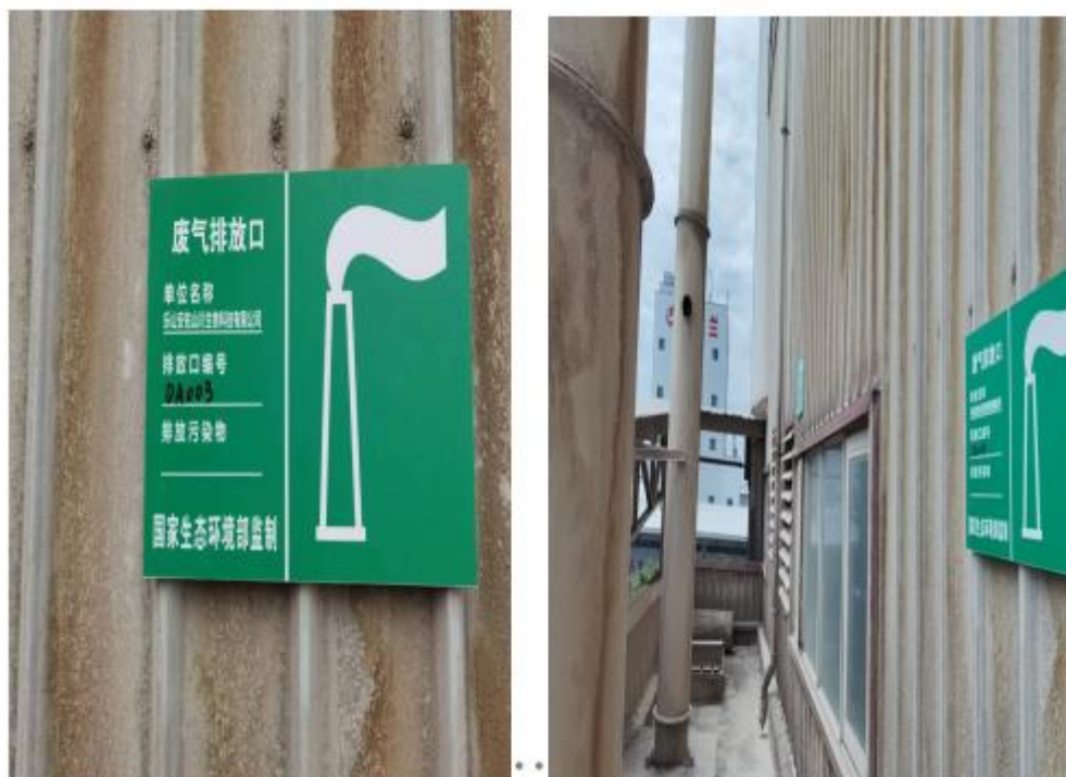
DA003.....DA003 废气治理设备
